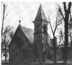
ST. STEPHEN'S CHURCH, STEUBENVILLE
